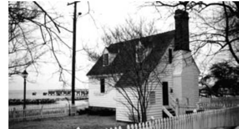
The Thomas Archer house and store burned in 1814, but was re-built in the 19th century on its original foundation, including a basement now used for wheel barrows and shovels. Rocks around the foundation are ballast from sailing ships.
