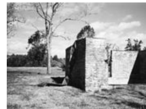
Isabel peeled off a portion of the copper cap from the lone standing building on Green Spring. A huge shag bark hickory tree in the background also fell victim to the hurricane.
